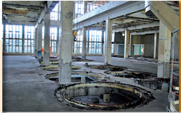
The cored building K90 in March 2017.
